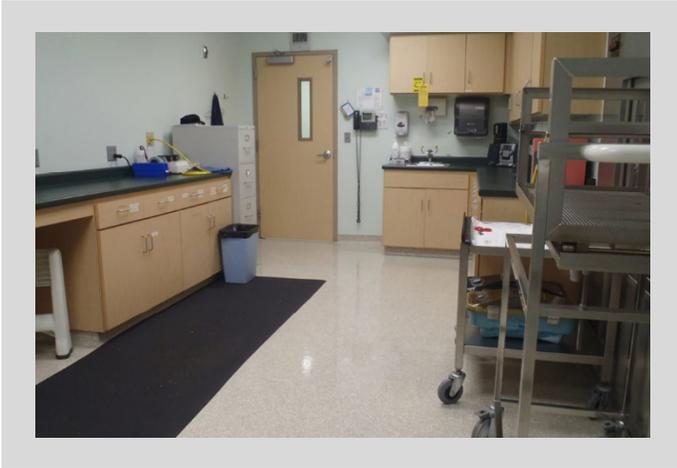
The system was coated and sealed using Peran STC and Flowseal UV. These low odor products deliver a durable and robust finish to the floor system, which provides chemical and abrasion resistance and a UV stable formulation to retain the color integrity of the floor finish.
