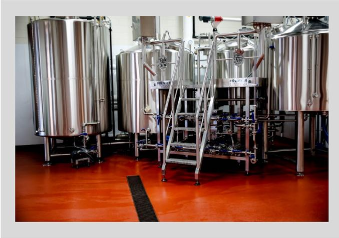
Approximately 2,500 sq. ft. of Flowfresh SL was quickly applied over three days in the new production area, bottling line and storage rooms. The antimicrobial system was installed with a full broadcast of aggregates to enhance its slip resistance. A topcoat of Flowfresh SR Sealer was applied to complete the dusky red floor finish.
