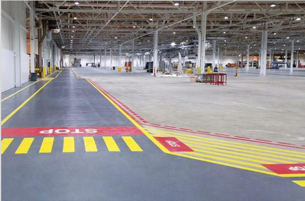
For the spaces that would be faced with more challenging demands, 40,000 square feet of the highly durable epoxy floor mortar Flowtex (1/4") was installed. This system has enhanced abrasion, wear, scratch and chemical resistance, making it suitable for even the most heavy-duty processing environments.
