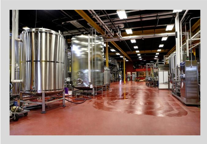
12,000 sq ft of Flowcrete's cementitious urethane floor system, Flowfresh SRQ was installed in a custom blend kitchen-red color within the main production and bottling area thanks to its antimicrobial, chemical resistant and hard-wearing properties.
