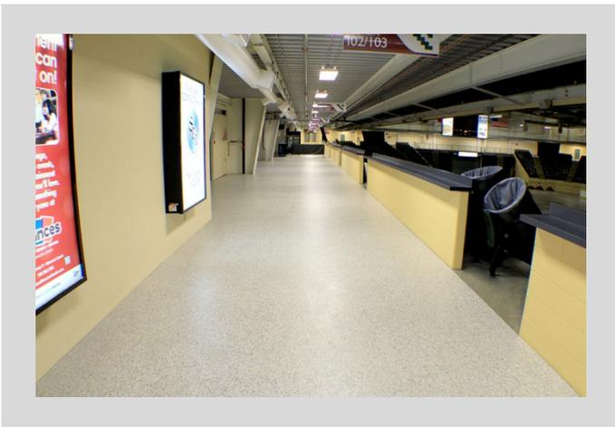
A methyl methacrylate (MMA) system, Flowfast Flakes cures just 60 minutes following application and is ideally suited to renovation or resurfacing projects on account of its ability to minimize downtime within live trading spaces.
