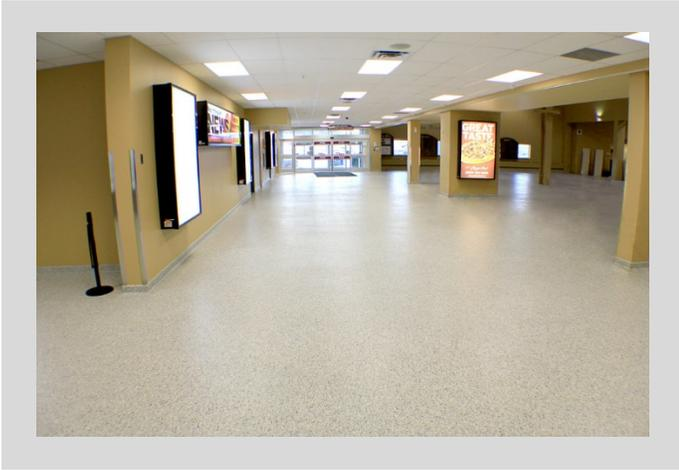
movements in the suspended slab. Combining Flowcretes' decorative, self-level and fast-cure Flowfast Flakes system, installed at 1/8", with a semi-flexible urethane body coat and semi-flexible top coat, the new system has performed incredibly well to date with not one single crack telegraphing through.
