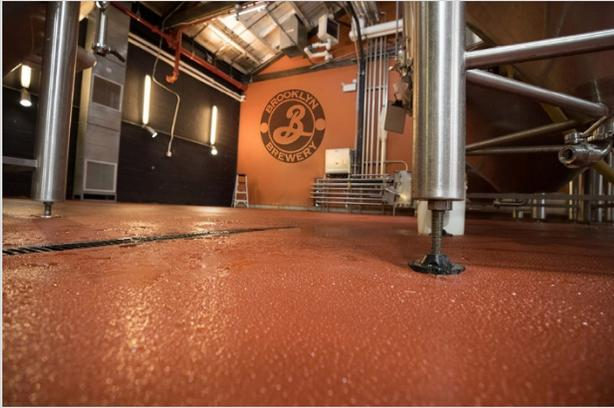
Flowfresh material is highly durable offering excellent thermal cycling and thermal shock resistance. This makes the material ideal for installation in areas subject to extremely hot temperatures or those that may be exposed to intermittent hot spillage or hot water wash down processes.
