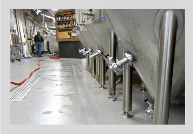
Flowcrete's antimicrobial treated cementitious urethane flooring system, Flowfresh SRQ was also installed over a smaller area at a heavy duty thickness of 1/4" to provide a positively textured floor finish, which is resistant to thermal shock and moisture vapor transmission.
