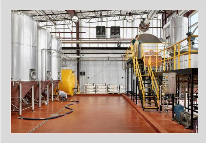
Flowfresh has been designed to be a key production line component, as its seamless, impervious and easy to clean finish minimizes the risk of contamination build up at floor level. In fact, Flowfresh's ability to create an ultra-hygienic surface led to the range achieving HACCP International certification. HACCP International helps reduce the threat of contamination incidents by providing the food and beverage industry with strict guidelines for building materials and equipment.
