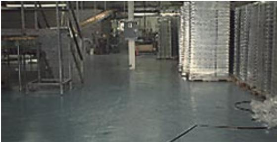
Worn, trowelled epoxy mortar in commercial bakery
